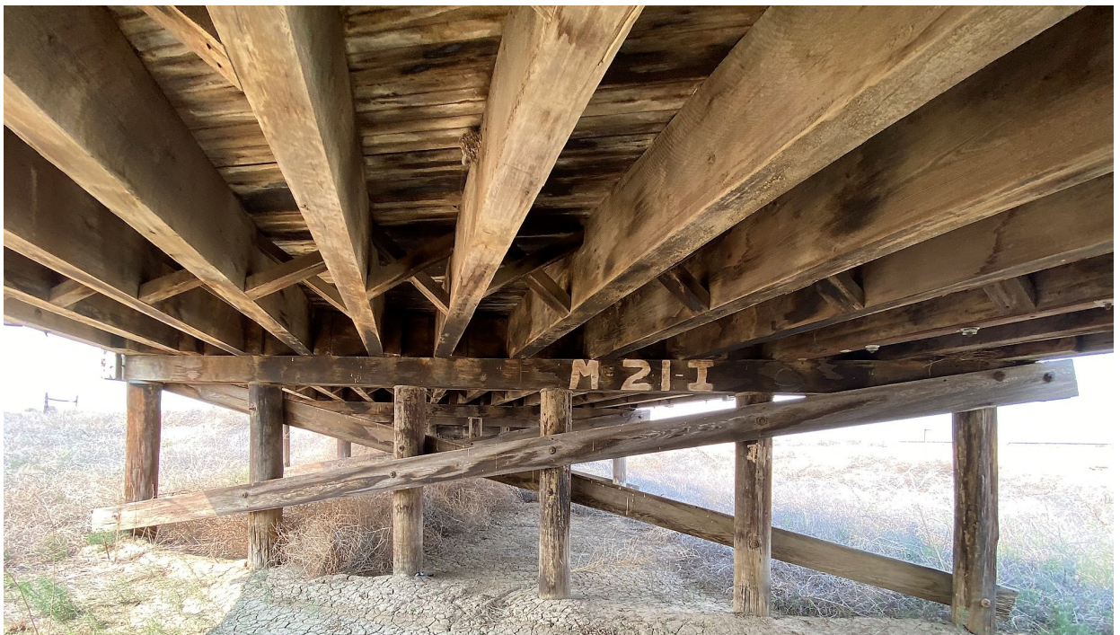
Photo 3 - Girders and Piles at Pier
