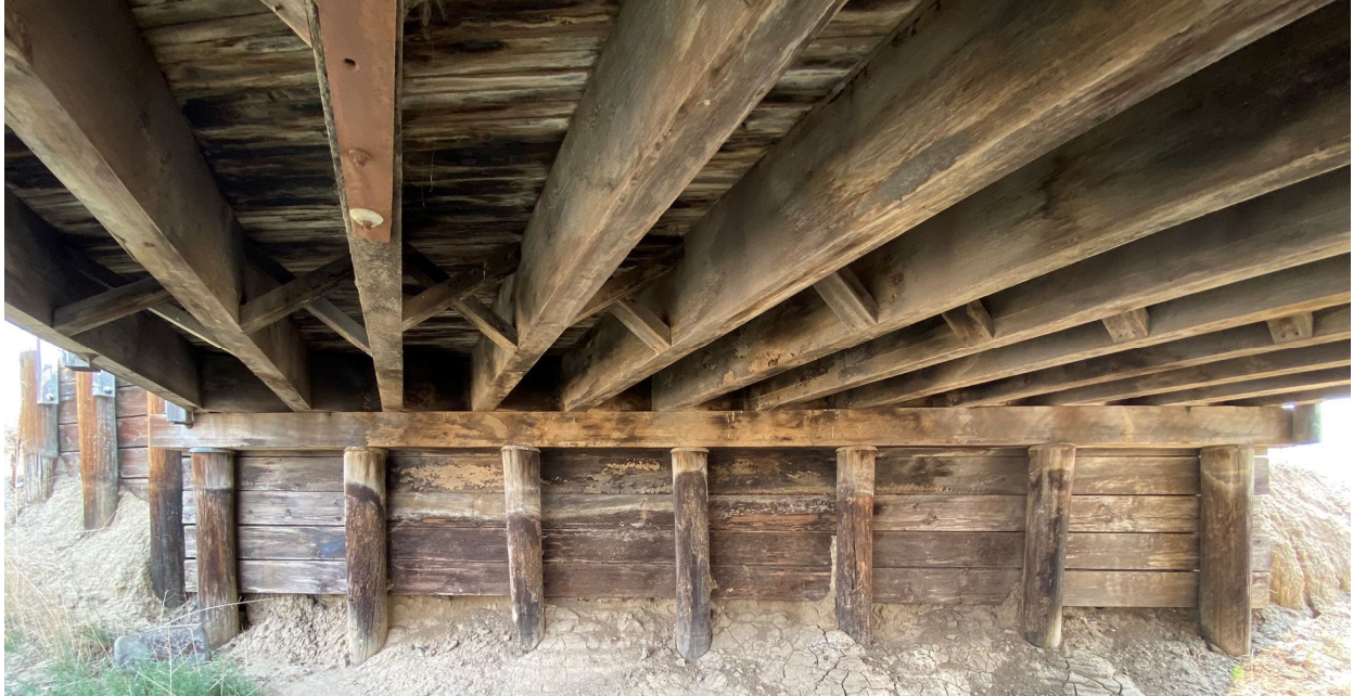
Photo 2 - Abutment and Repaired Girder
